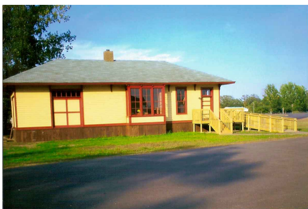
THE NEW STONE LAKE DEPOT/MUSEUM
