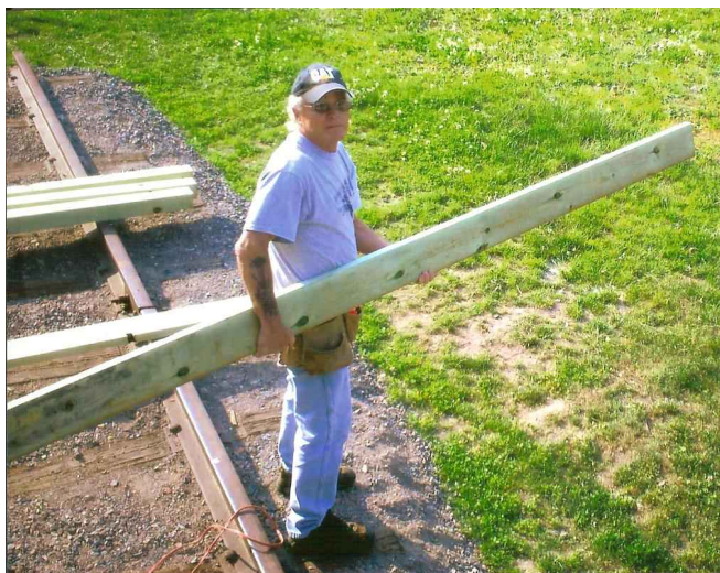
Jim Young begins work on the entrance platform to the caboose
